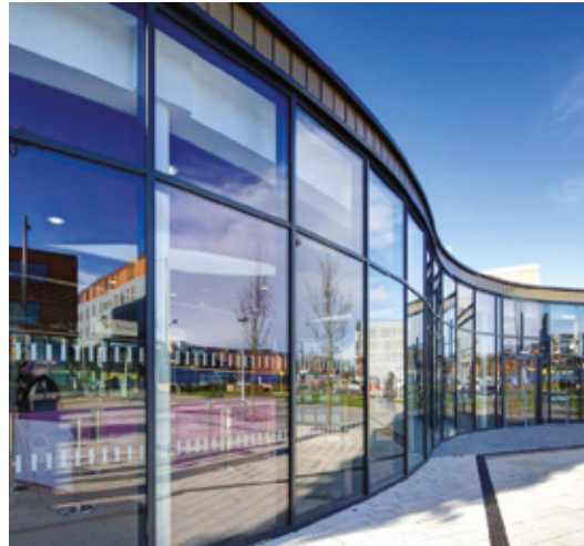
Figure 5.6: Wakefield Westgate station after redevelopment Source: Wakefield First
