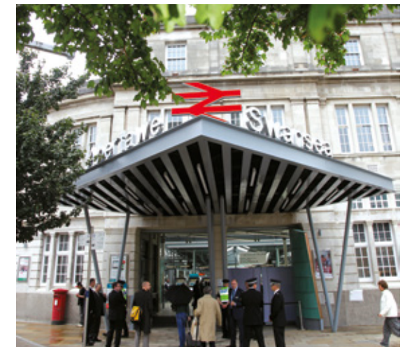
Figure 5.5: Swansea station concourse after redevelopment Source: South Wales Evening Post
